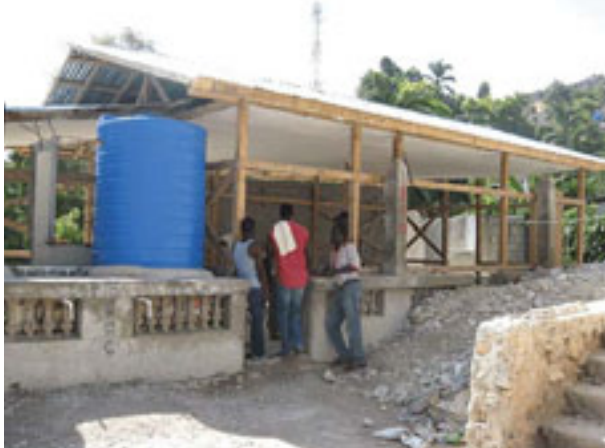
Our Lutheran Church being rebuilt – Carrefour
